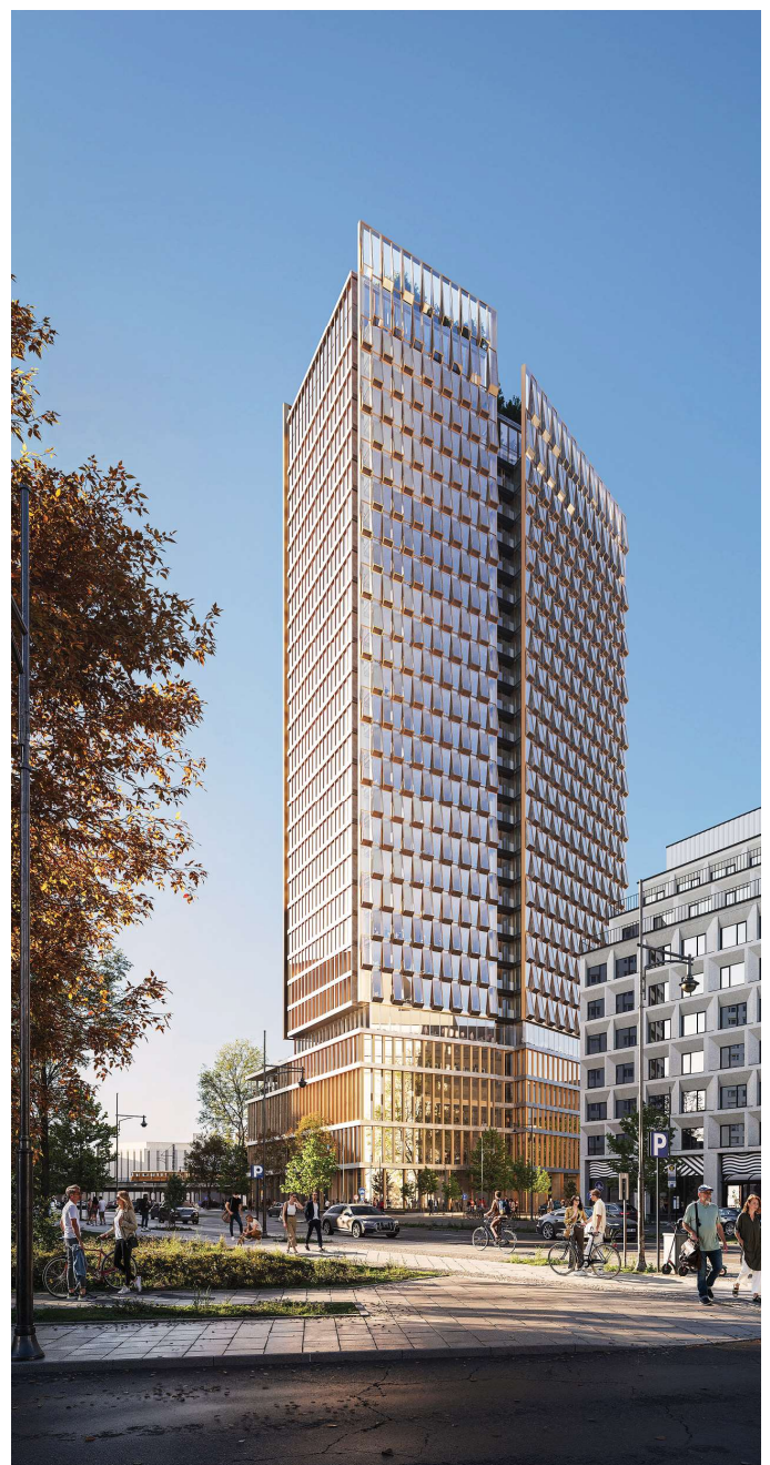
The building is composed of a base, a body and a crown
